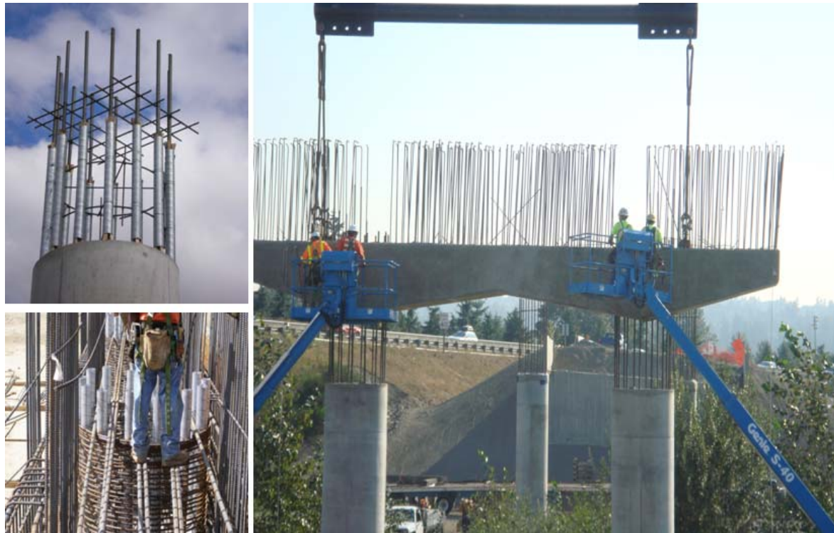
FIG. 9: PRECAST BENT CAP UNDER CONSTRUCTION IN WASHINGTON STATE
