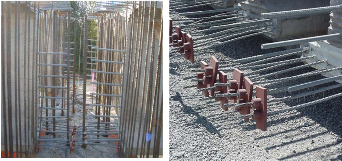
FIG. 4: STRAND ANCHORS AT MOMENT RESISTANT CONNECTIONS
