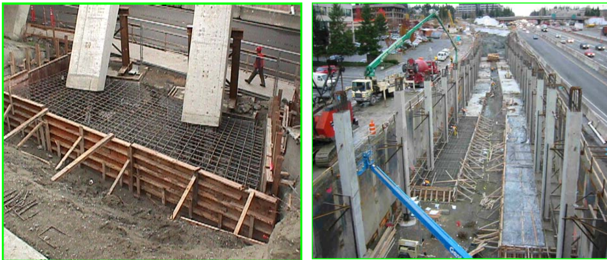
FIG. 6: PRECAST COLUMNS ON SPREAD FOOTING
